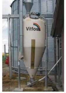
Segregation was observed in big bags and in polyester silos, whereas no segregation was observed in fibreglass silos.
