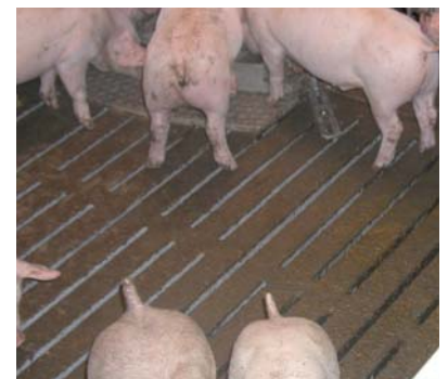
Pen with bristle concrete slatted floor in the dunging area.
