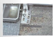
*Corrosion of slatted floor in a pen floor treated with an impregnation product.*
