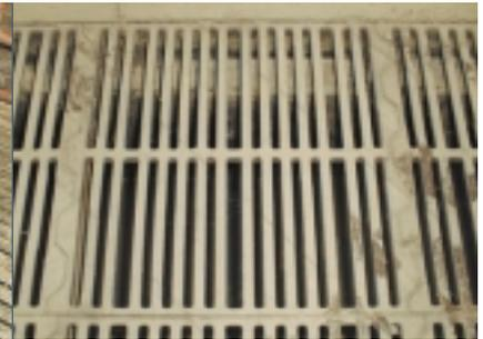
The cast iron floor has a 12 mm plate form and 12 mm slit, however every 5 slit is 20 mm.
