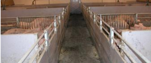
Solid floor in inspection alleys
