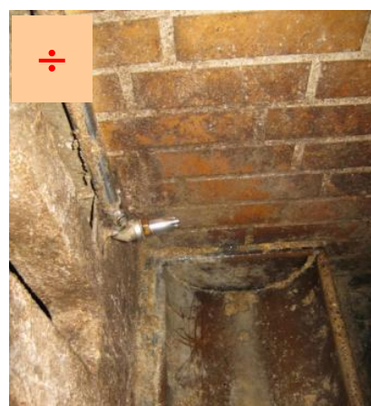
A simple method for flushing of pipes
