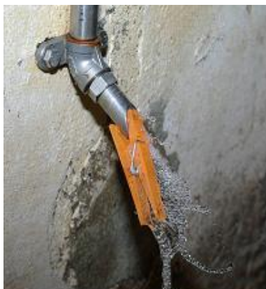
A simple method for flushing of pipes
