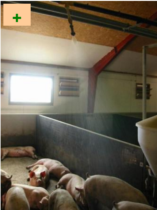
Sprinkling with flat nozzles placed correctly
