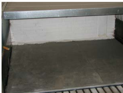
Rubber mat fastened to a countersunk rail.
