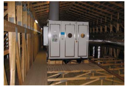
Biological air purifier from SKOV A/S called Farm AirClean-BIO 3U.
