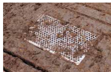
The manure hatch must be installed close to the nesting areas. When lying areas are cleaned daily, manure is pushed directly into the slurry pit.
