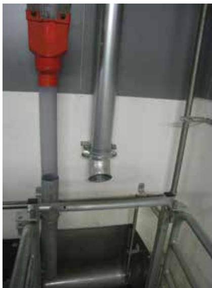
Trough valve: the air is directed towards the head of the sow.
