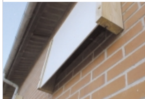
The wind shielding with adjustable inlet area typically has two or three options for adjustment. With three options, adjustment during the summer must have a light area corresponding to the inlet area of the valve, spring/autumn adjustment must reduce the light area to 50%, and winter adjustment must reduce the light area to 25% of the inlet area of the valve.
