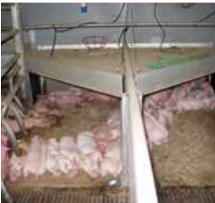
The Aniheater is placed below the cover (left-hand side). E-heat is installed in the cover (right-hand side).
