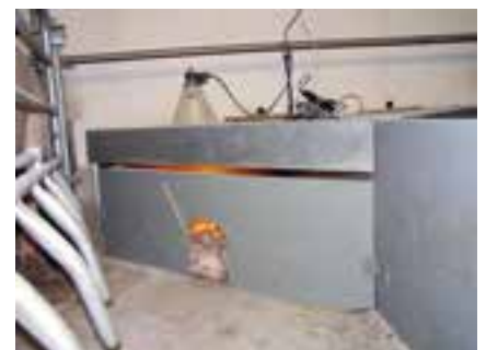
Creep area covered by a board the first few days post-farrowing. Ventilation in the creep is ensured by an opening between the upper front edge and the board.
