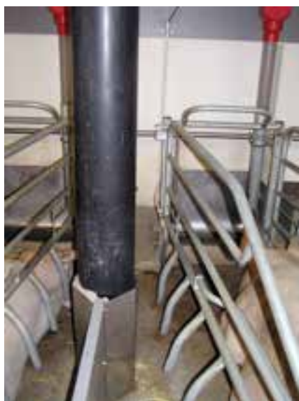
Point extraction in a farrowing facility with partly solid floor.
